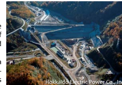
Kyogoku Power Plant, HEPCO
